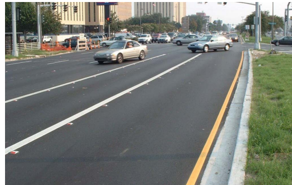
Pavement after GlasGrid installation
